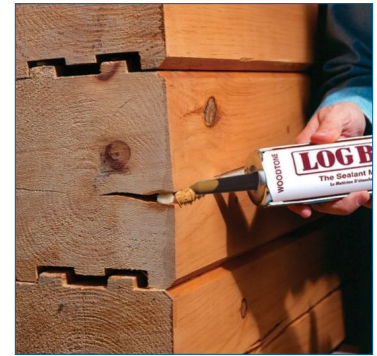
EXAMPLE: Chinking Sealant for cracks.
