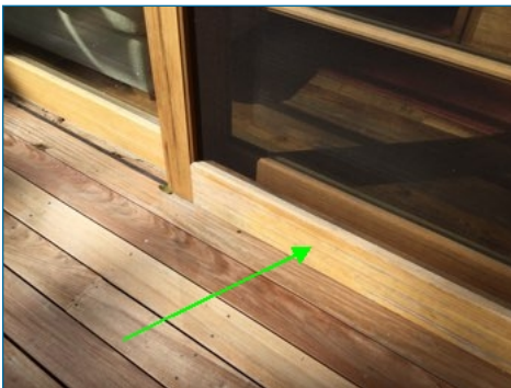
South facing doors window and sliders need to be resealed with coating due to heavy sun exposure. Have doors and slider frames treated and sealed to preserved during routine maintenance.
