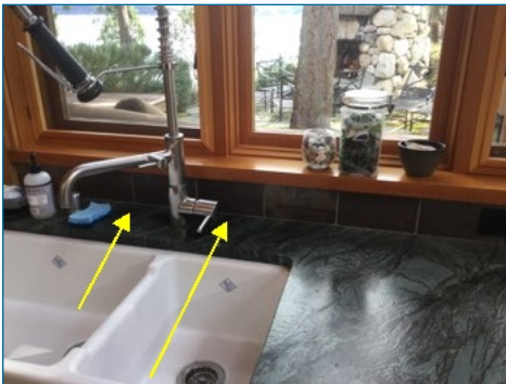
Caulk back splash where grout or caulk is missing. Noted behind main sink.
