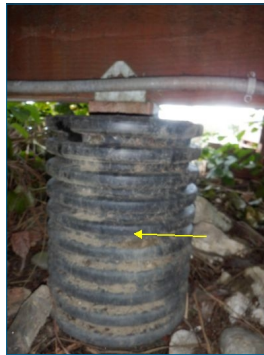
Remove Plastic forms below concrete.
