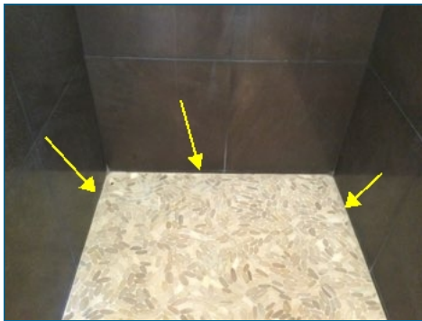
Caulk floor at base of shower where needed to prevent water intrusion under flooring.
